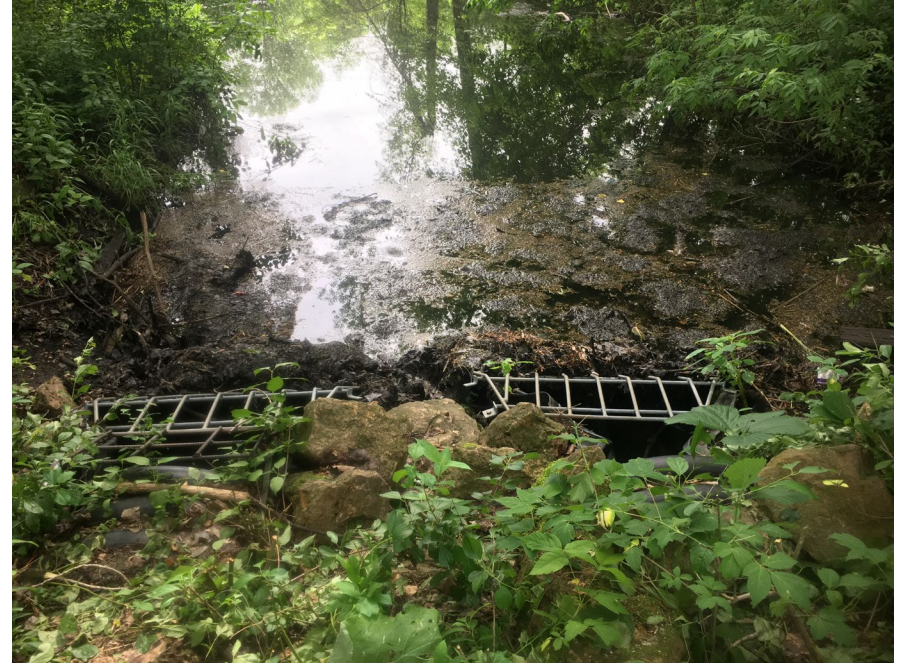
Upstream side of culvert
