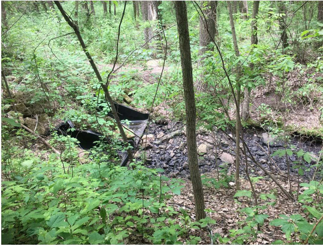
Double culvert that is dry until rain events
